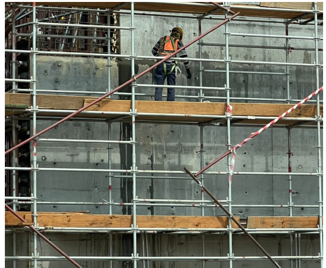
Temporary access and site works
