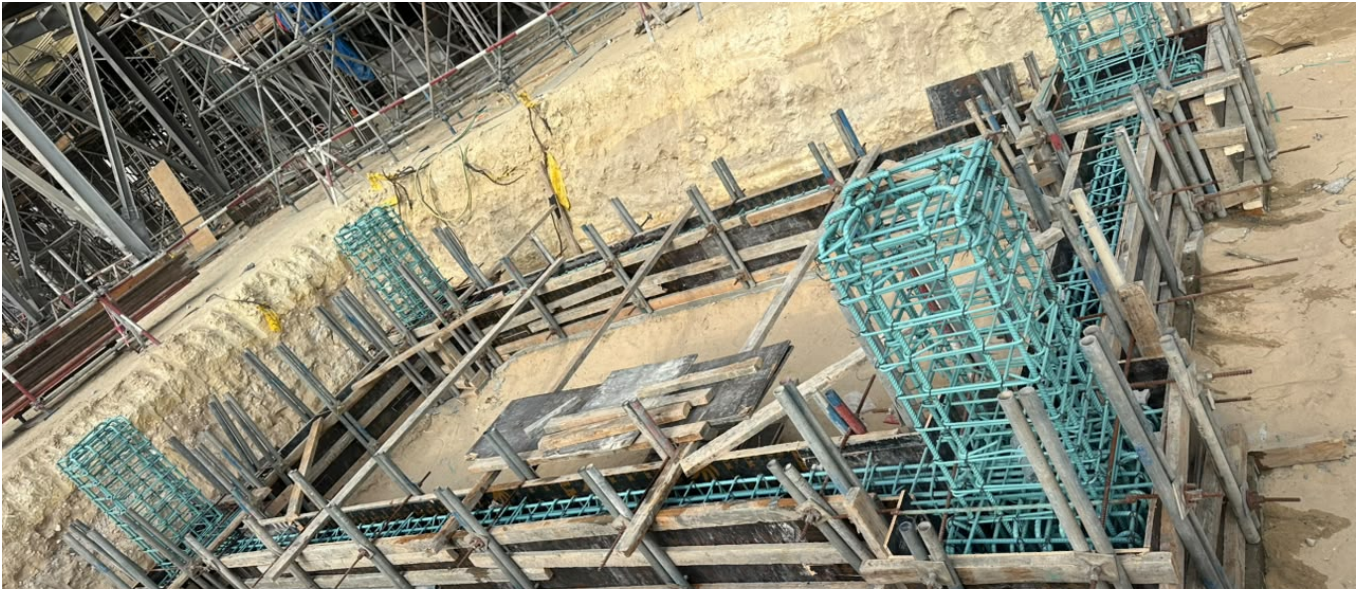
Supplied site photograph: reinforcement and foundation formwork.
