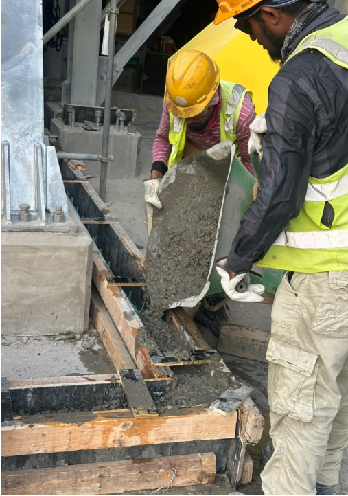
Concrete placement at a foundation.
