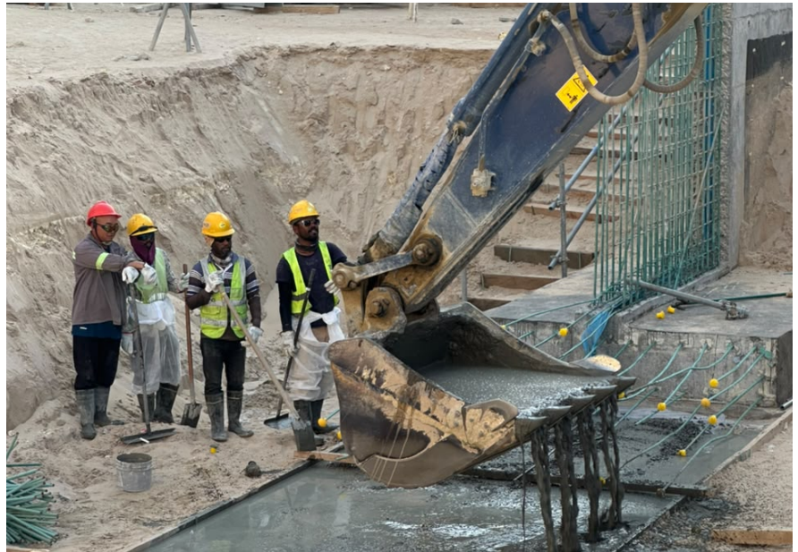
Excavation and concrete placement activity.
