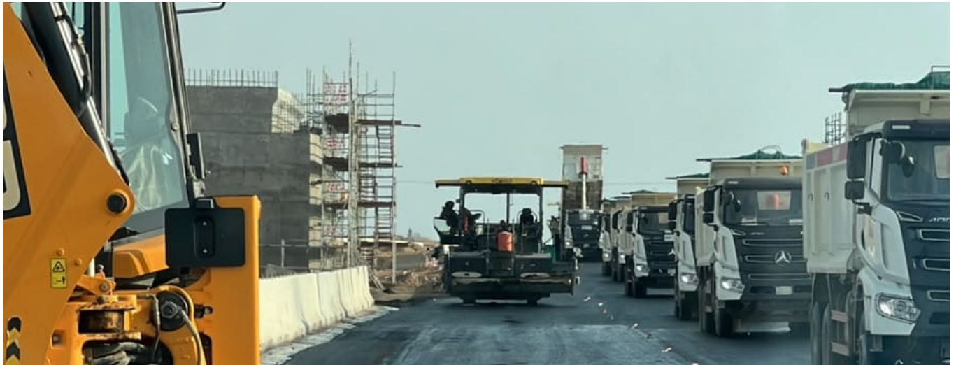
Supplied image of site vehicles and roadwork equipment.
