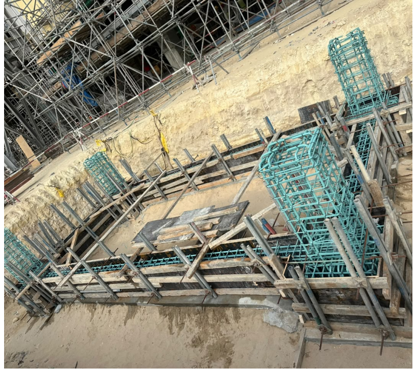
Reinforcement and formwork.
