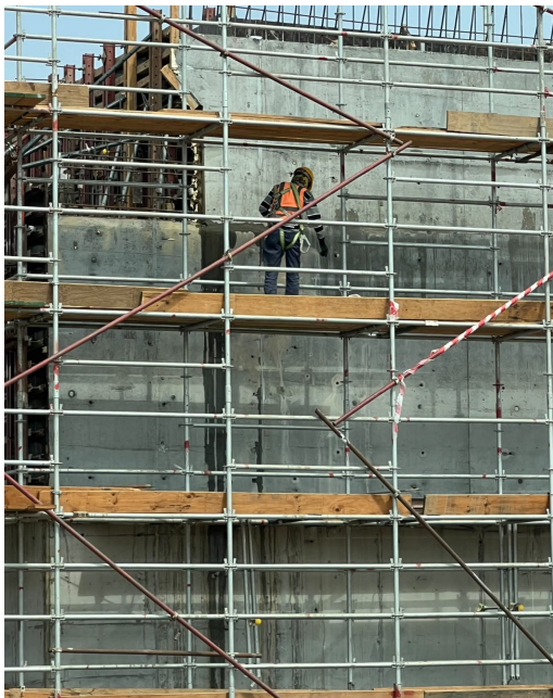
Temporary access at a concrete structure.
