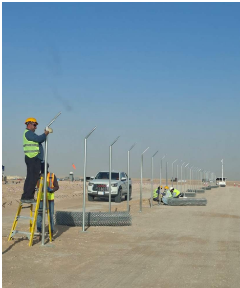
Site setting-out and alignment.
